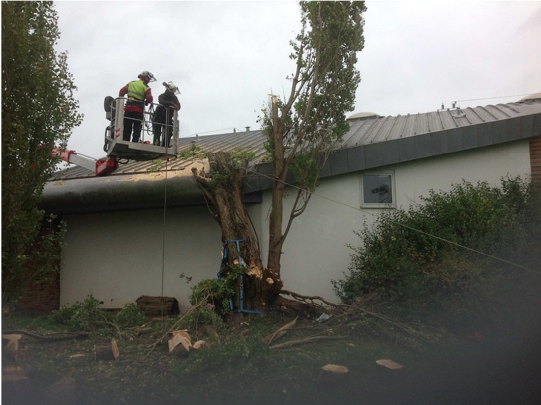
Figure 1: Dismantling operation on poplar following the St Jude's Storm.
